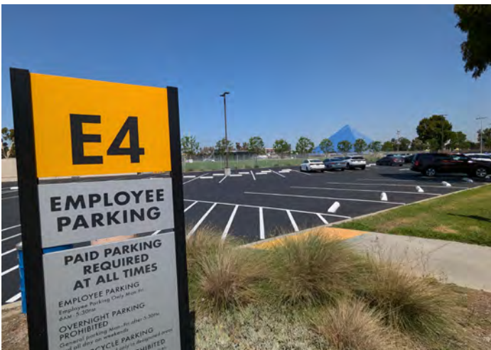
Repair, reslurry, and restripe Lot E4.
