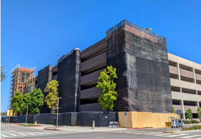
Brick facade removal, resurface, and internal repairs to all 3 parking structures.
