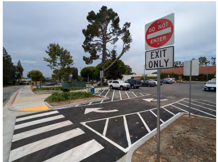
New vehicle exit added to Lot E10.
