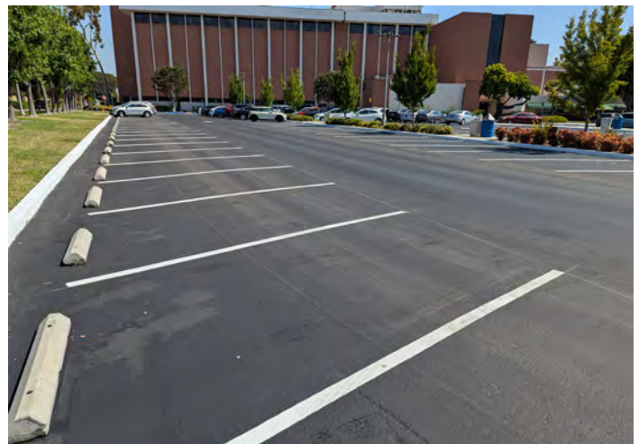
Repair, reslurry, and restripe Lot E9.
