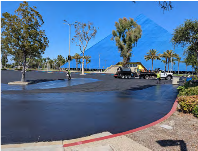
Repair, reslurry, and restripe G11.
