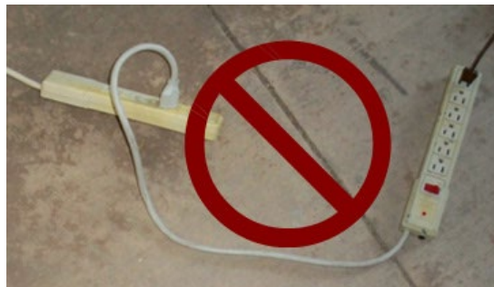
Not OK: daisy chain with 2 power strips
