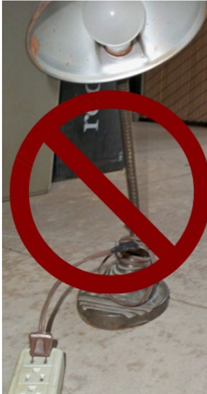
Not OK: metal to wire lamp on wet concrete
